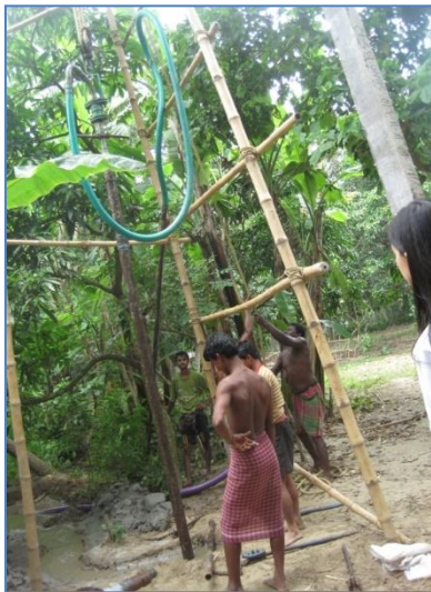
Figure 7: Bamboo scaffolding
