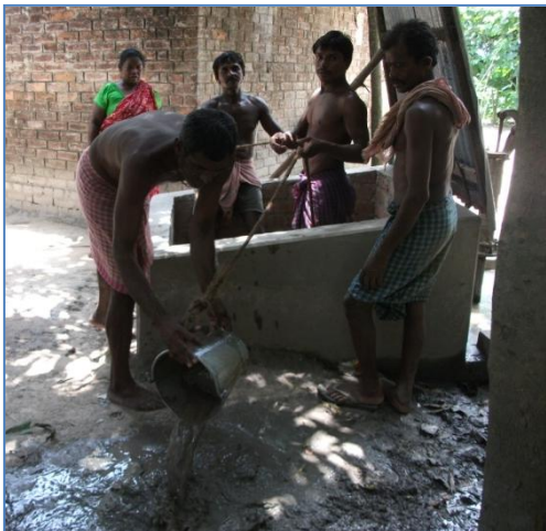
Figure 19: Dredging in progress
