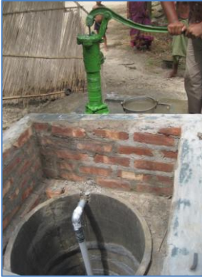
Figure 16: The delivery pipe
