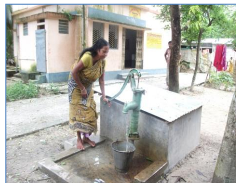
Figure 5: Bore-dugwell with handpump
