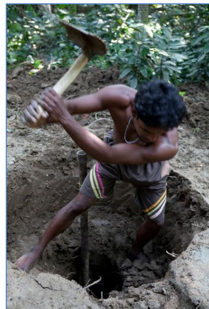
Figure 14: Digging from the top cutting around the inserted pipe
