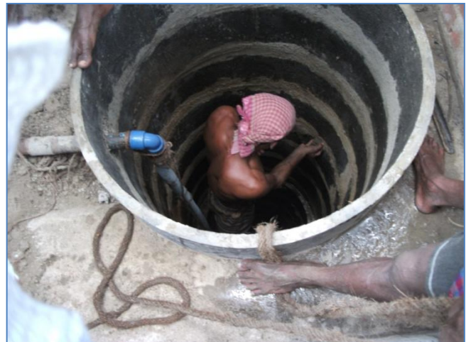
Figure 20: Repairing an old dugwell
