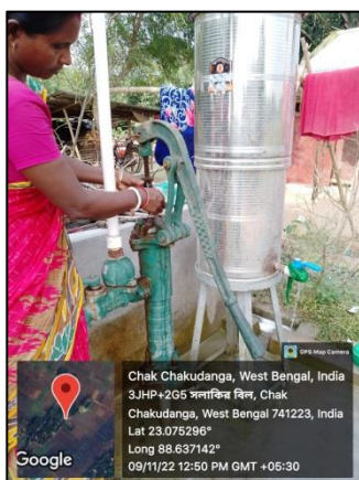
Figure 10: Maintenance of PW365 in Chakdah
