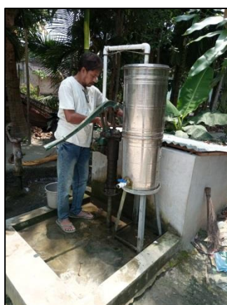
Figure 11: PW 358 filter maintenance in Swarupnagar
