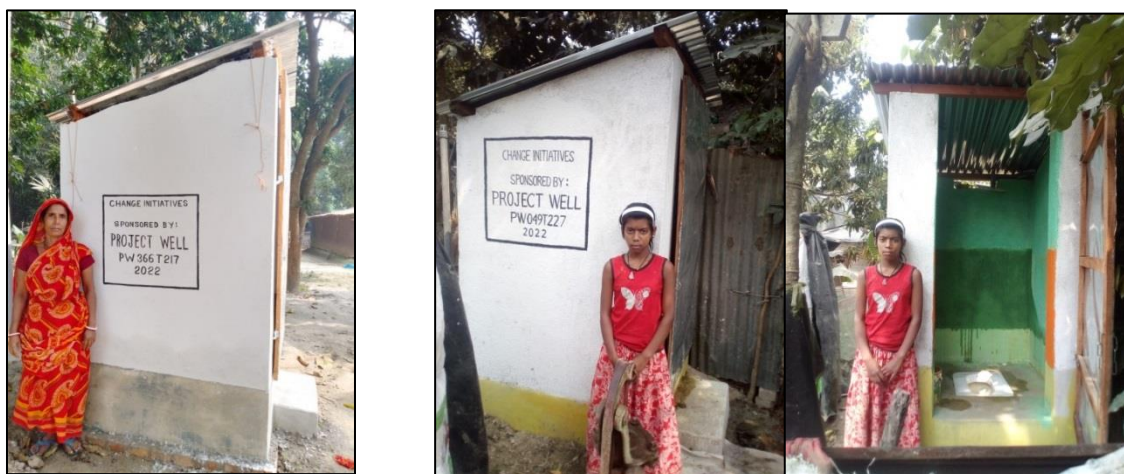
Figure 8: Toilet PW49T227_Kamdebkathi, Deganga
