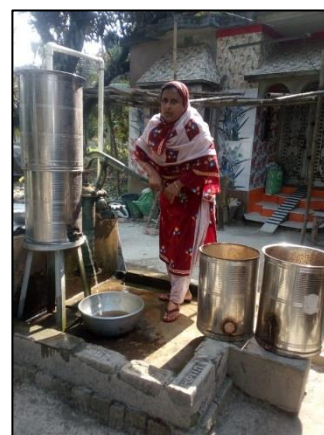
Figure 12: PW207_Replacement of the filter drums on 22nd Nov 2022
