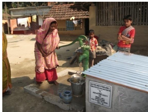
A newly constructed bore-dugwell # PW206.
