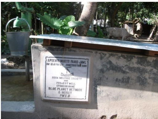
A newly constructed bore-dugwell # PW182.
